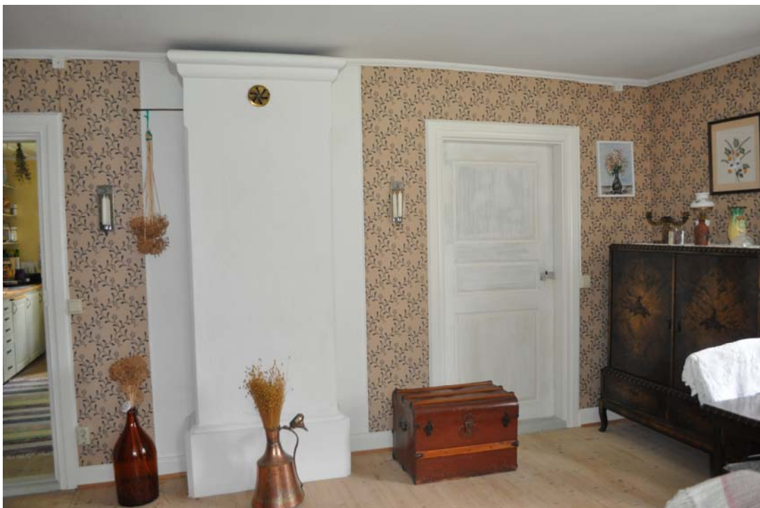
Livingroom with poor mans stove still in use. The flue gas from the kitchen stove is lead in channels inside the brickwork to take care of the heat and store it for the nights
